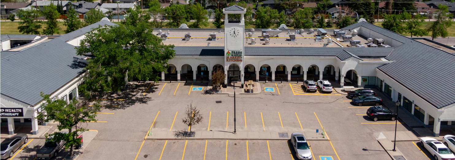
Building D - South Side
