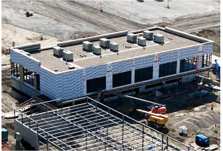
BUILDING D - POSSESSION - NOVEMBER 2026
