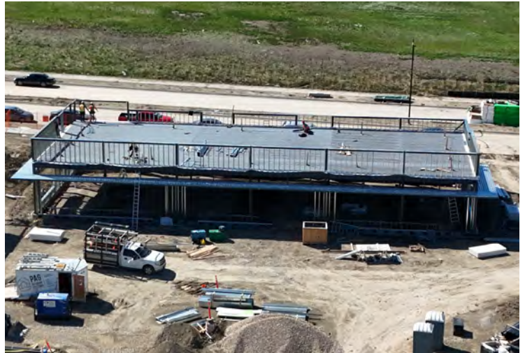
BUILDING F - POSSESSION - DECEMBER 2026
