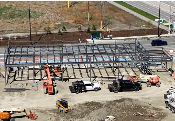
BUILDING J - POSSESSION - NOVEMBER 2026
