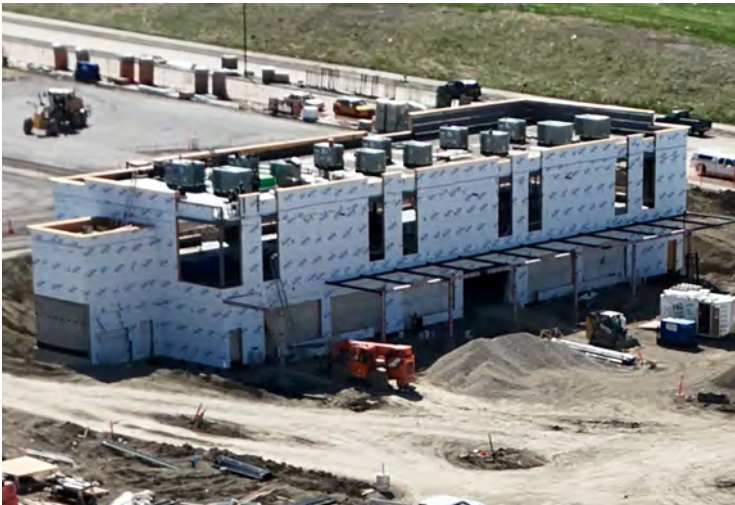
BUILDING E - POSSESSION - DECEMBER 2026
