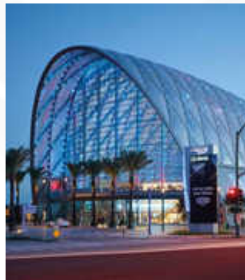
ARTIC (ANAHEIM REGIONAL TRANSPORTATION INTERMODAL CENTER)
