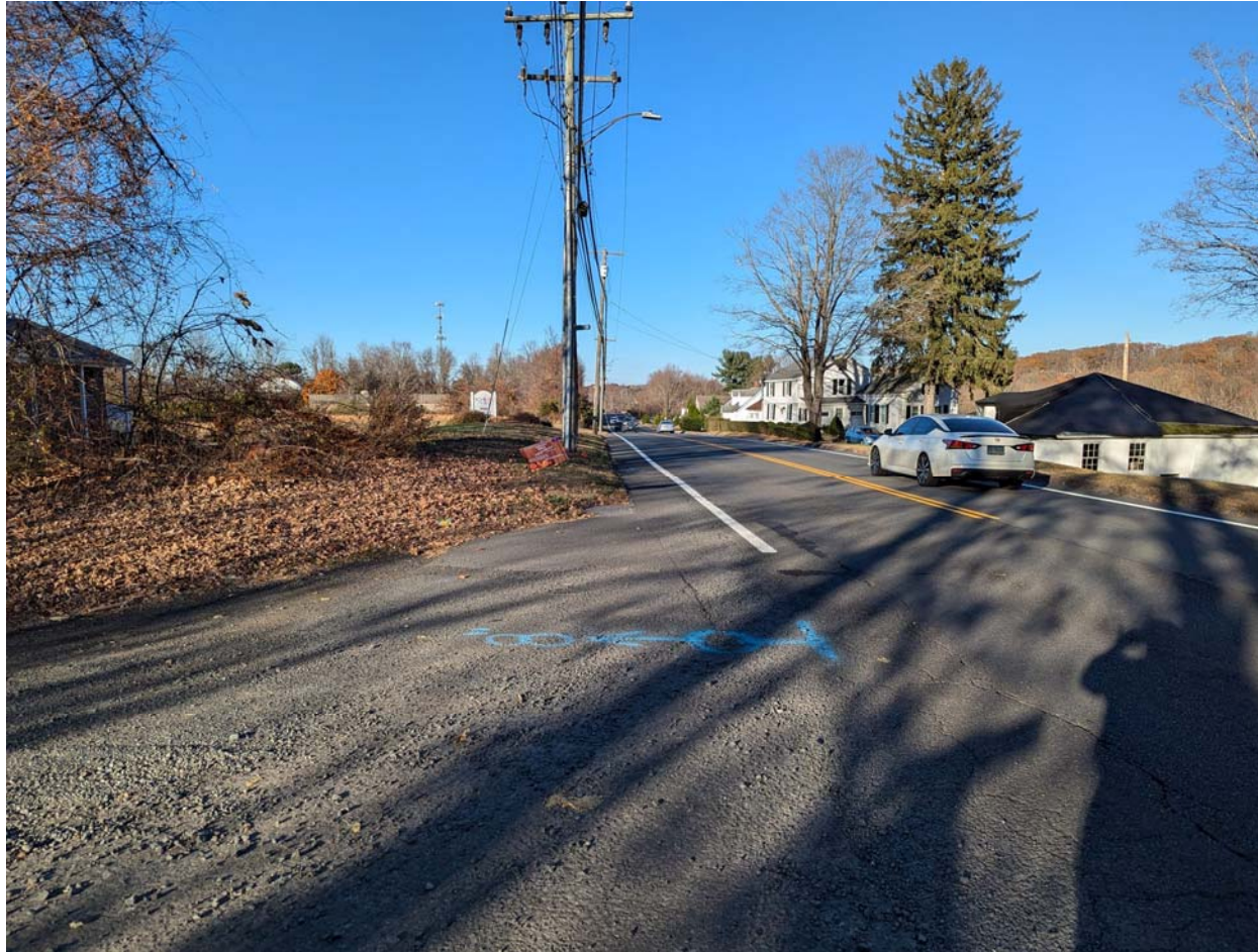
Entry Road, Trigo Drive View South Along Route 17/South Main Street
