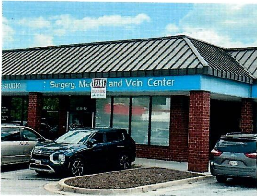
Glass storefront & Signage
