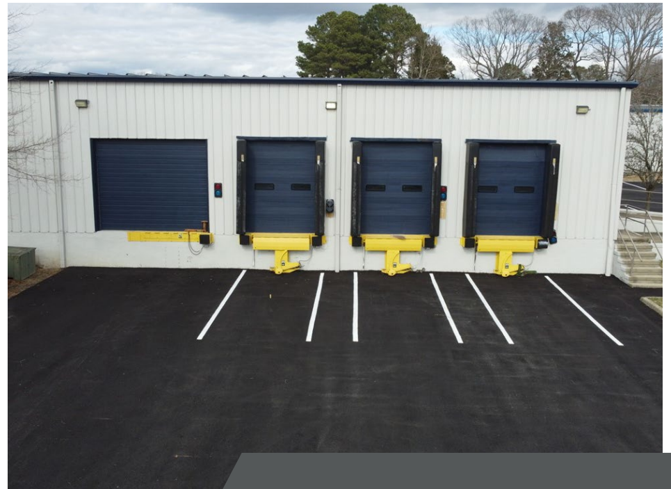
CANDLE FACTORY BUILDING 7521 RICHMOND RD., WILLIAMSBURG, VA
