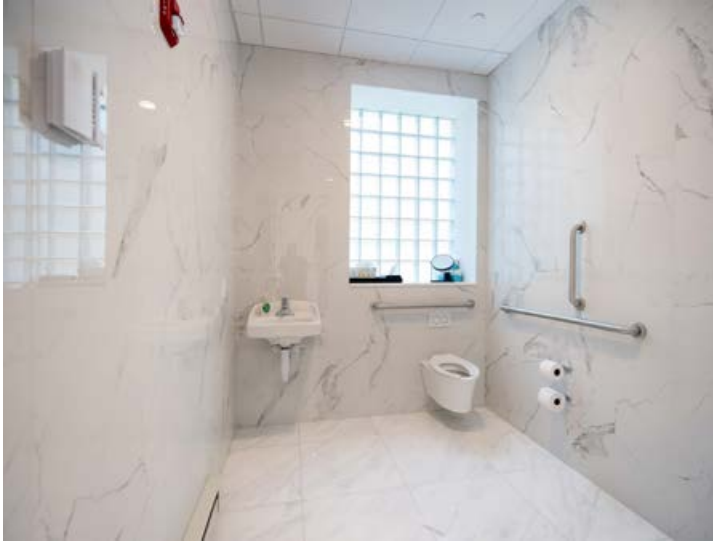
2nd Floor Bathroom
