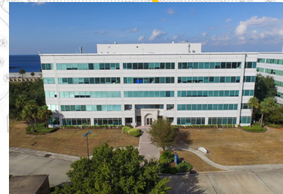
INFORMATION AND TECHNOLOGY CENTER #1 (ITC-1)
