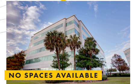
INFORMATION AND TECHNOLOGY CENTER #2 (ITC-2)
