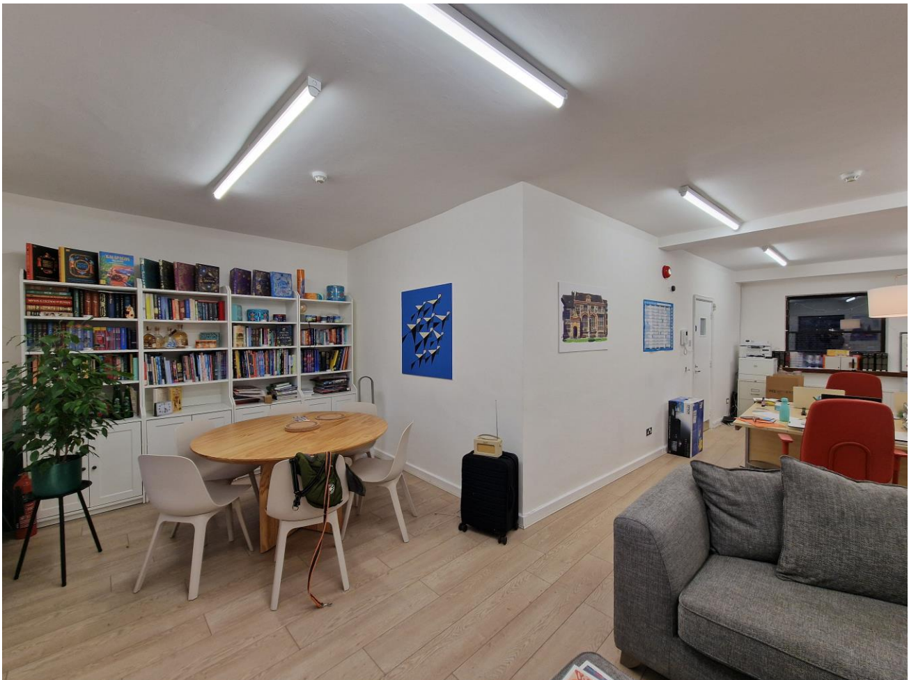
Space being refurbished. Photos of 4 th floor.
