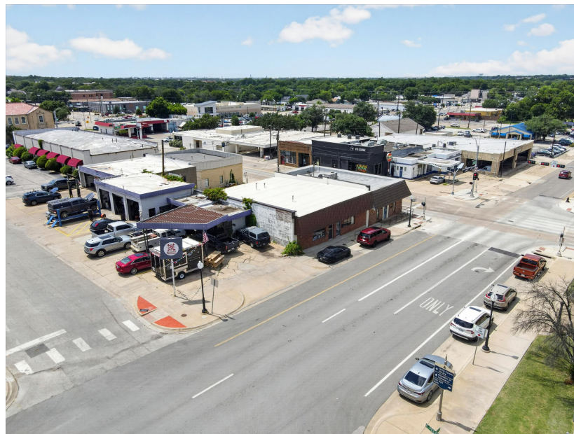
Aerial perspective — property visible at lower center; Downtown Square in background.
