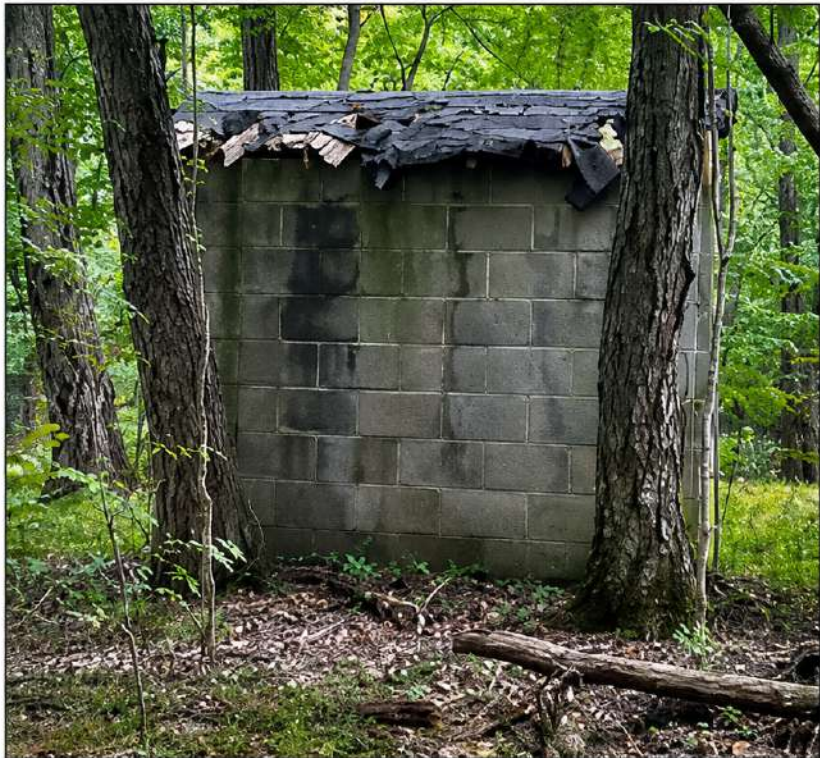
A - 4 Rear view of outbound structure.
