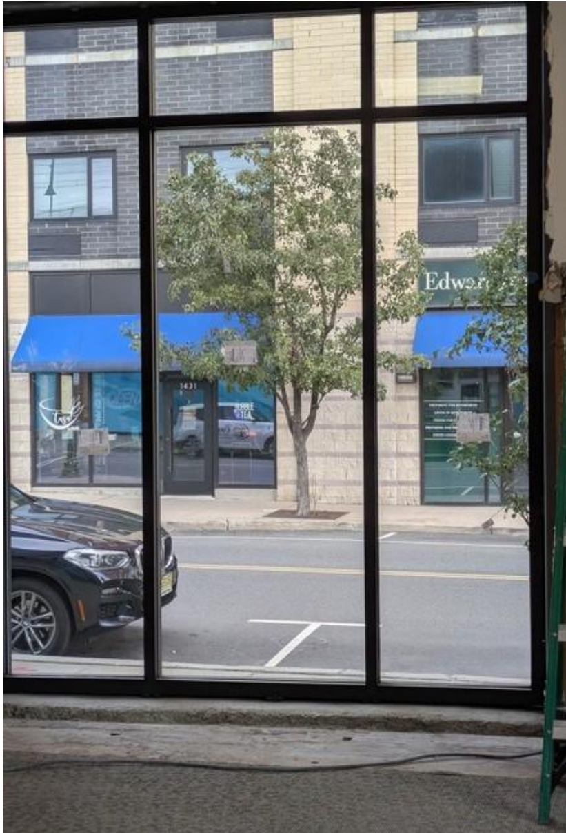
installed 8 x 6 windows facing Irving Street
