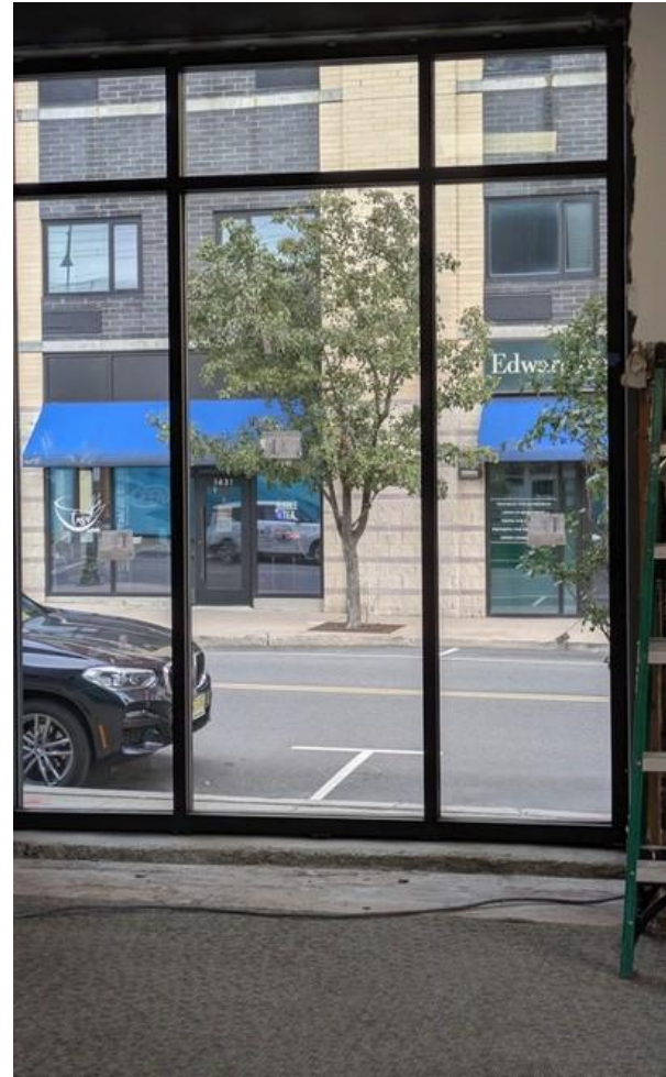
installed 8 x 6 windows facing Irving Street
