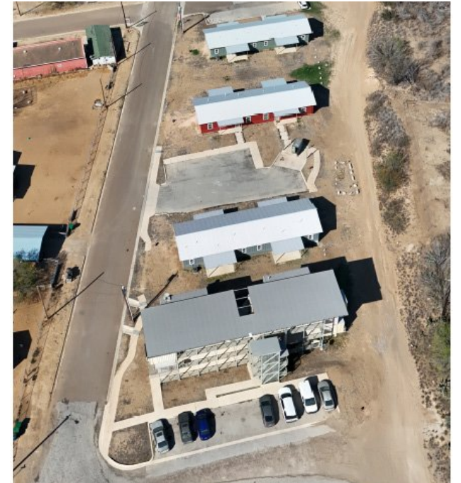
Aerial — the four buildings and on-site parking
