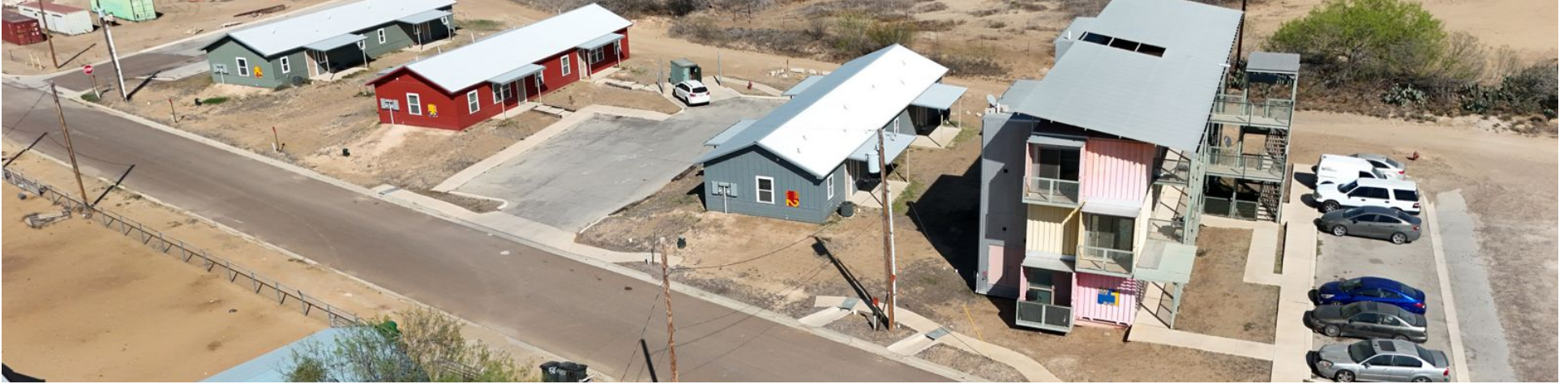
Buildings 2–4 (2025 duplexes, remodeled July 2026) and Building 1, along Berry Street
