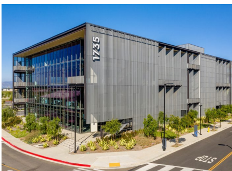
Building Street View
