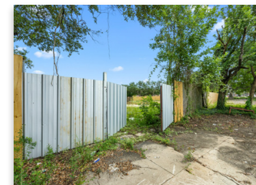
West-boundary fencing and the remnant concrete slab.
