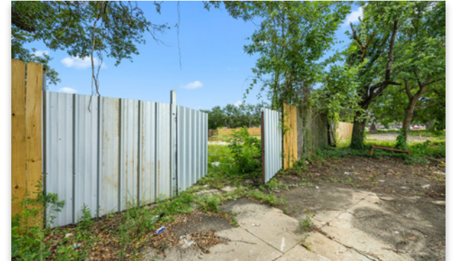
West boundary fencing and the existing concrete slab
