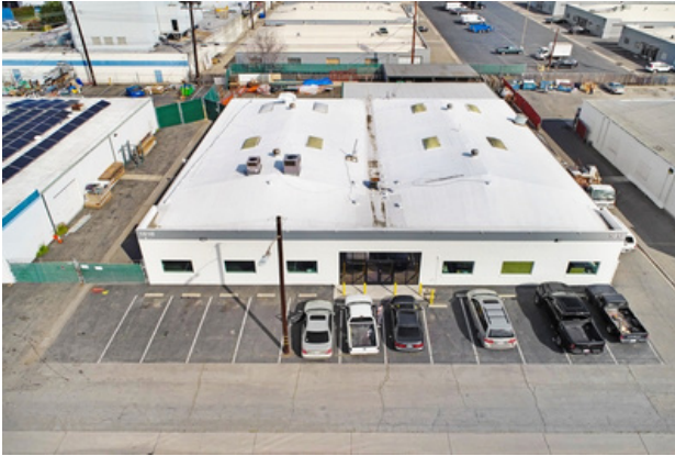
FRONT OF BUILDING
