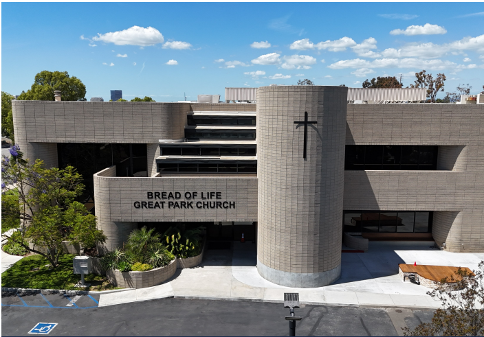
AERIAL VIEW — BUILDING & PARKING
