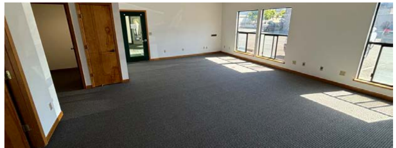
RECEPTION / FRONT ROOM WITH STOREFRONT GLAZING
