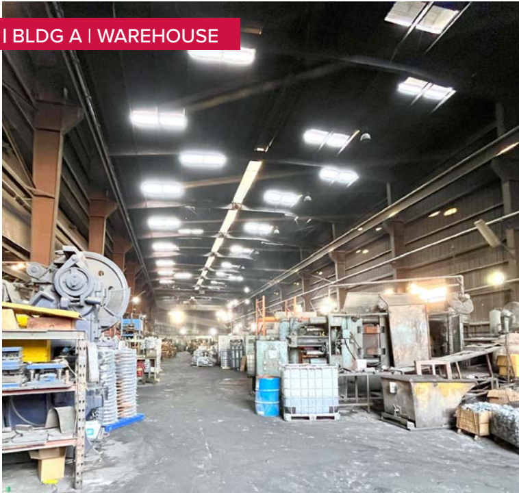
I BLDG A | WAREHOUSE CRANES
