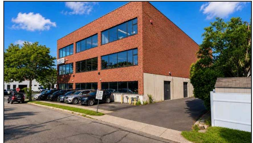
TWO DRIVE-IN DOORS ACCESSIBLE FROM BERKELEY ROAD
