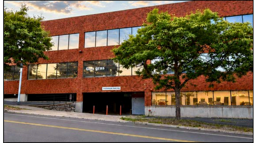
ENTRANCE TO 9,456 SF DRIVE-THRU GARAGE WITH PARKING FOR 25 CARS
