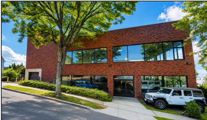
SHOWROOM ENTRANCE & DRIVE-IN DOOR ON MARLBOROUGH TERRACE
