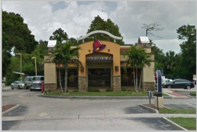
Taco Bell - Renovated 2017
