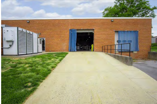
View of Drive In Door
