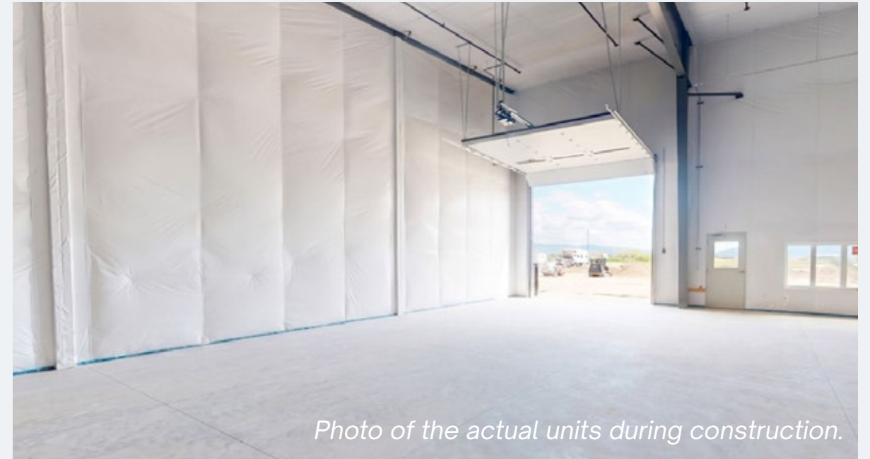
Photo of the actual units during construction.
