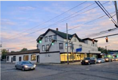
Front of Structure - Corner view of signalized Diamond Hill road (left) as it meets Social Street.
