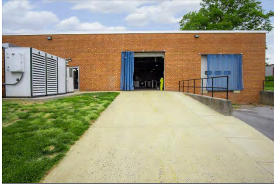
View of Drive In Door
