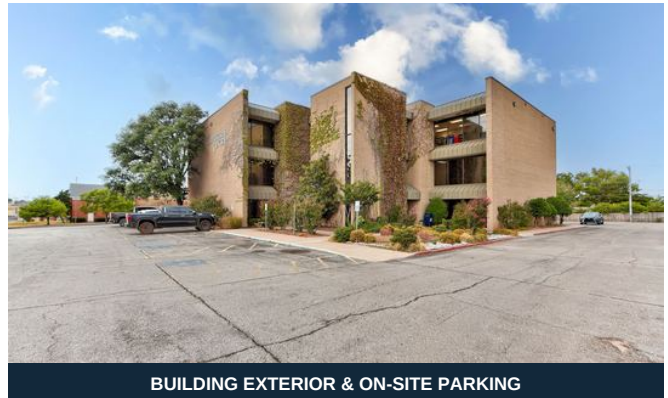
BUILDING EXTERIOR & ON-SITE PARKING
