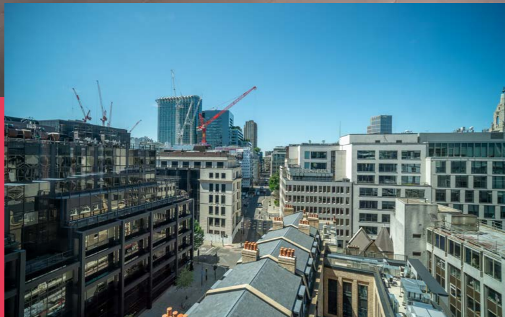
Photograph from Level 6 office looking West to Finsbury Square.
