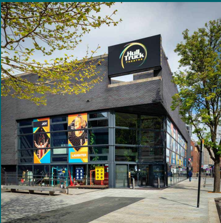
Hull Truck Theatre
