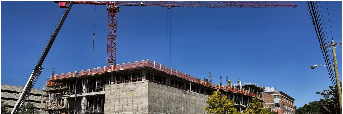
Active construction at the Carilion / VTC district adjacent to the property
