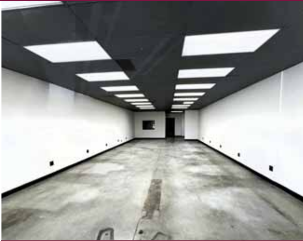
4750 Almaden Expressway, Suite 144 Interior
