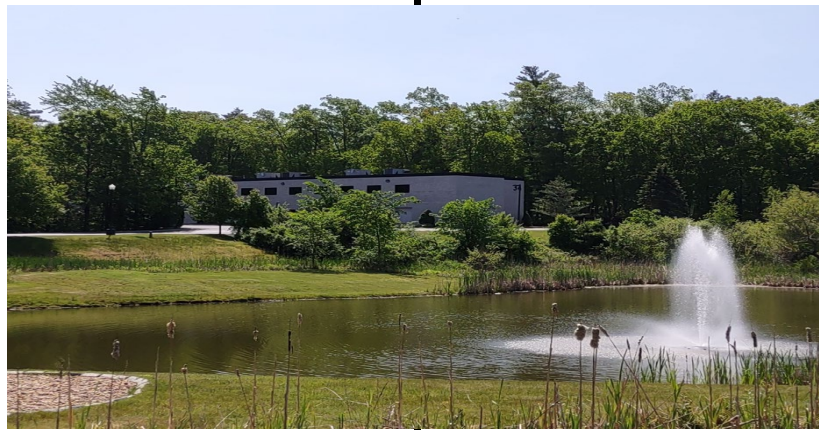
Rear of facility
