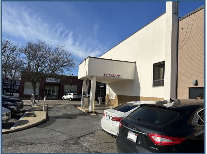
Former Bank Drive-thru
