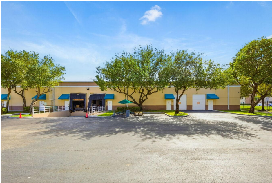
Rear Elevation — Loading Docks, Drive-In Doors & Truck Court
