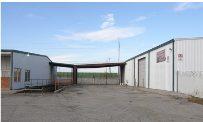
Shared Dock Well/Courtyard Loading
