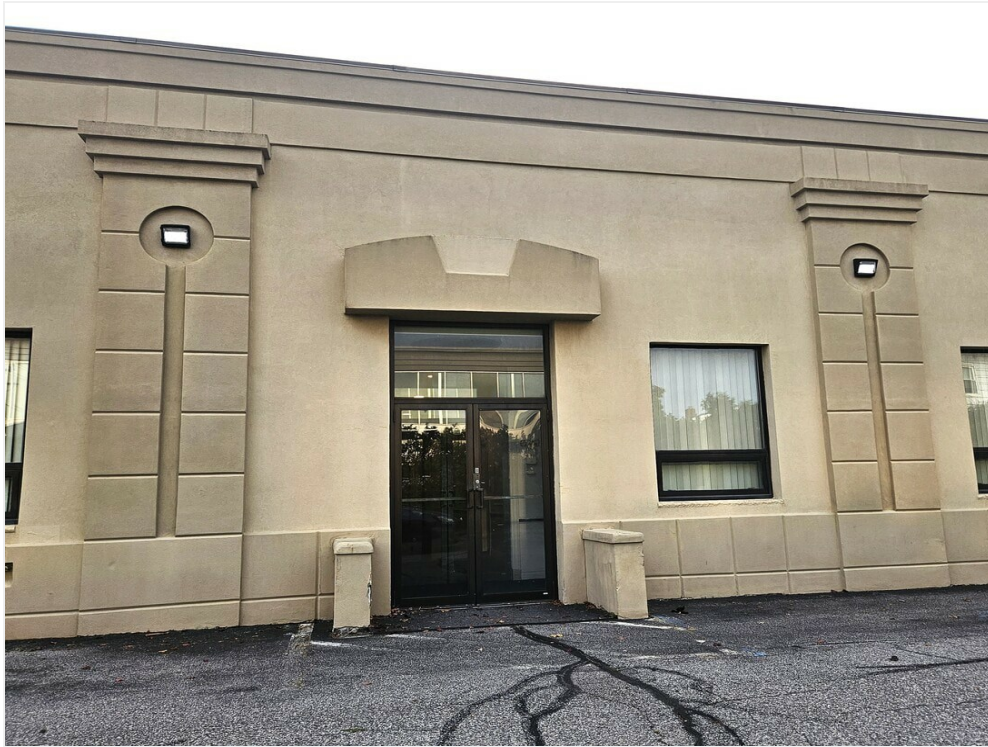
Rear Entry from Parking
