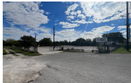
1.5 ACRE OF BASE MATERIAL/ASPHALT
