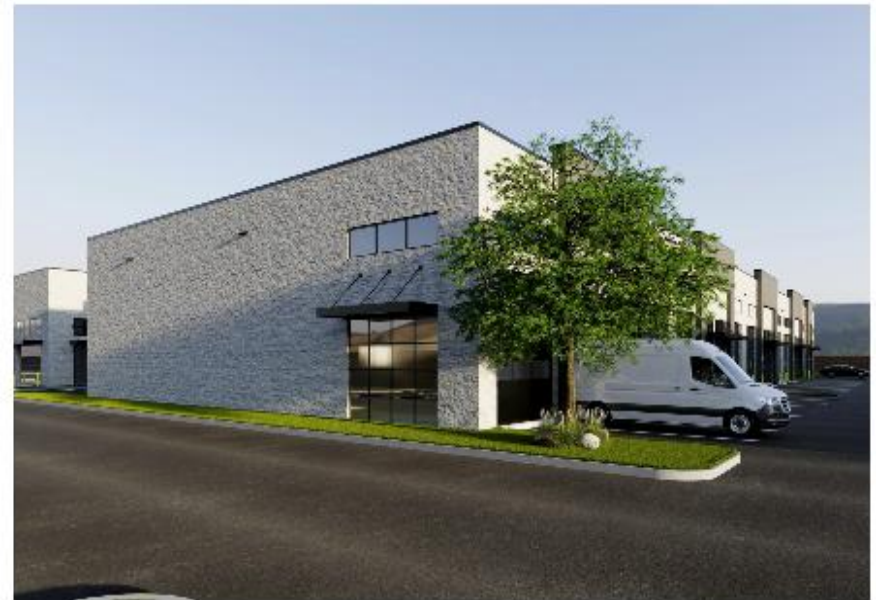
FLEX BUILDING SIDE VIEW
