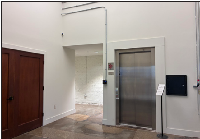
Common Area Elevator
