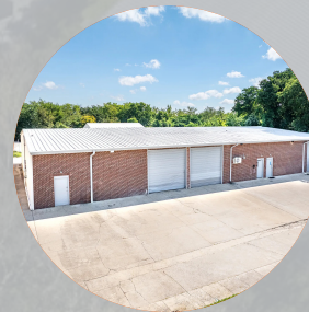
FRONT & REAR DRIVE-IN DOORS
