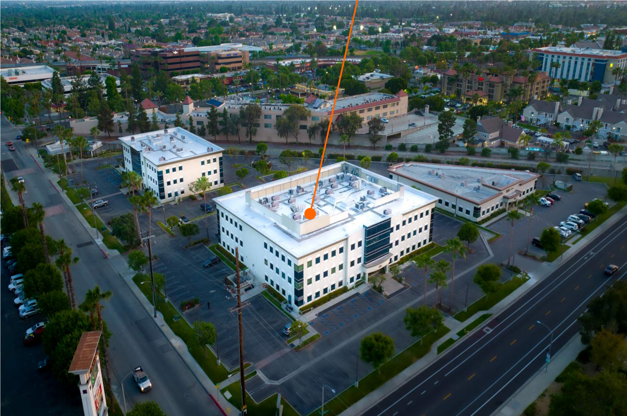
488 EAST SANTA CLARA BUILDING
