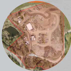
LOCATED TO SERVE WA & ID
