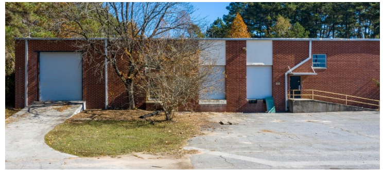
DRIVE-IN RAMP, DOCK & PAVED YARD
