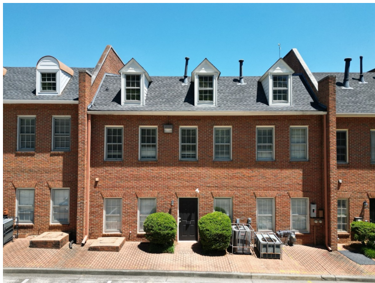
Rear elevation — secondary access and additional parking
