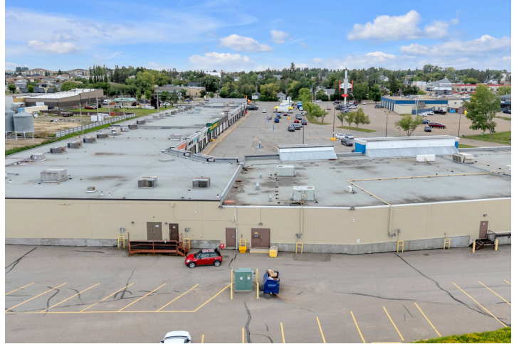
Rear Building Access + Parking
