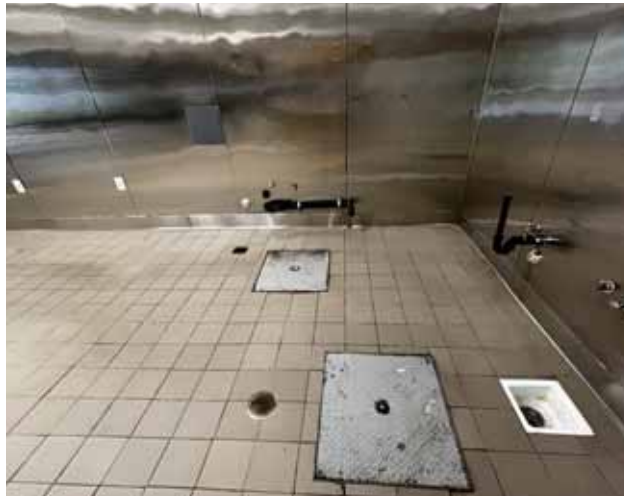
Plumbing Stub Outs | Inground Grease Interceptors
