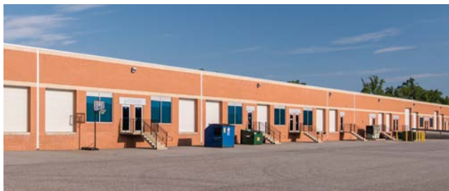
Flex/R&D dock and drive-in loading
