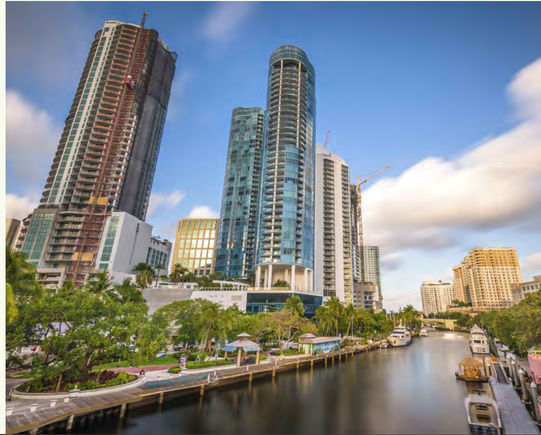
Situated along the Riverwalk
