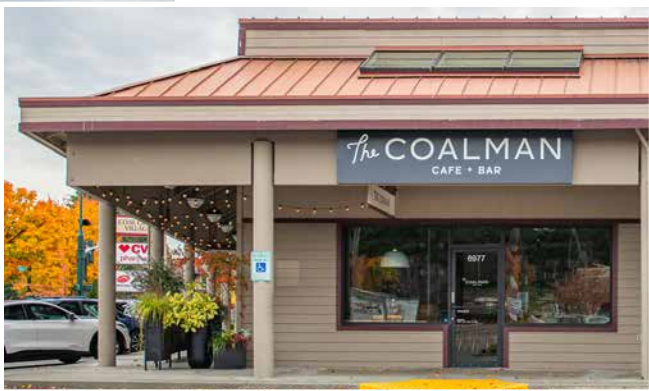
West Corner View on Coal Creek Parkway
