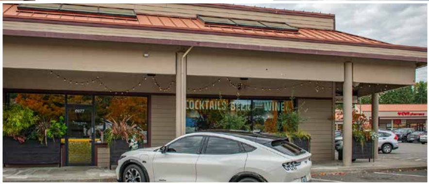
North Corner View on Coal Creek Parkway
