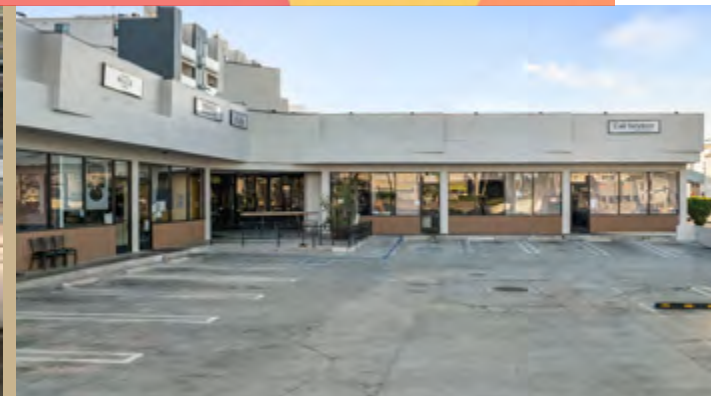
10020-10036 Venice Blvd, Culver City, California
