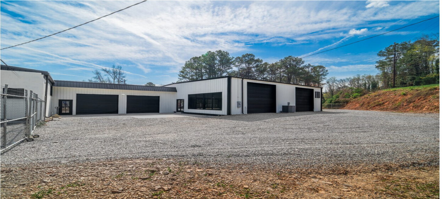
Shop / Warehouse Elevation with Multiple Roll-Up Doors
